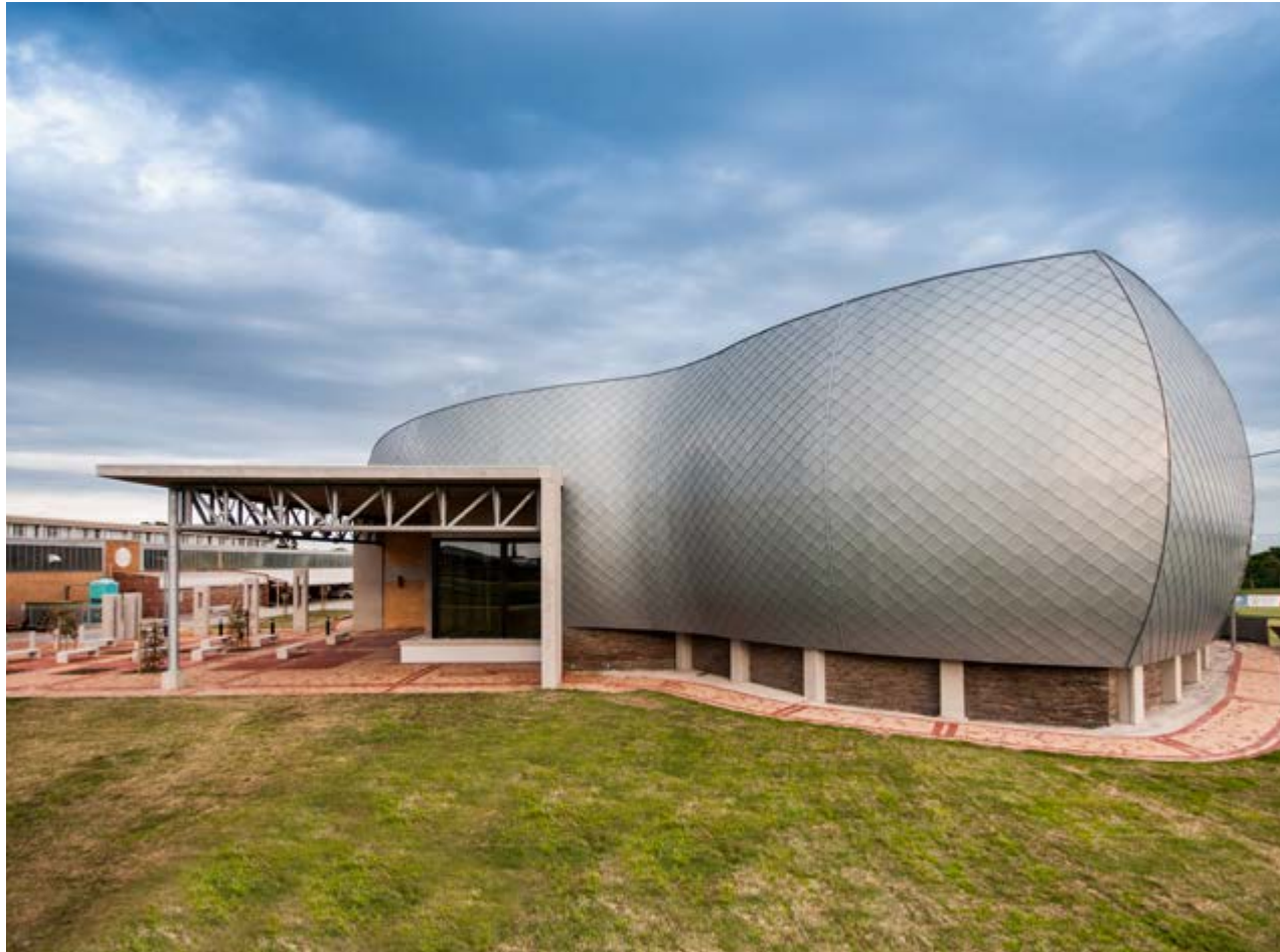
Nelson Mandela University's New Engineering Building, Phase I.
